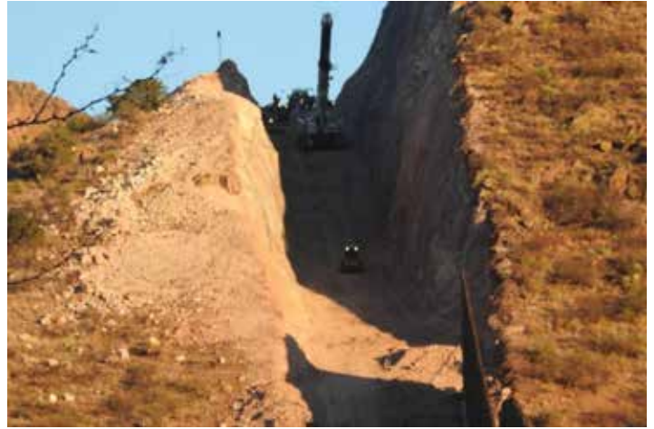
Sheer cliffs blasted into Guadalupe Canyon. Jan. 8, 2021. 31.33834, -109.0922.
