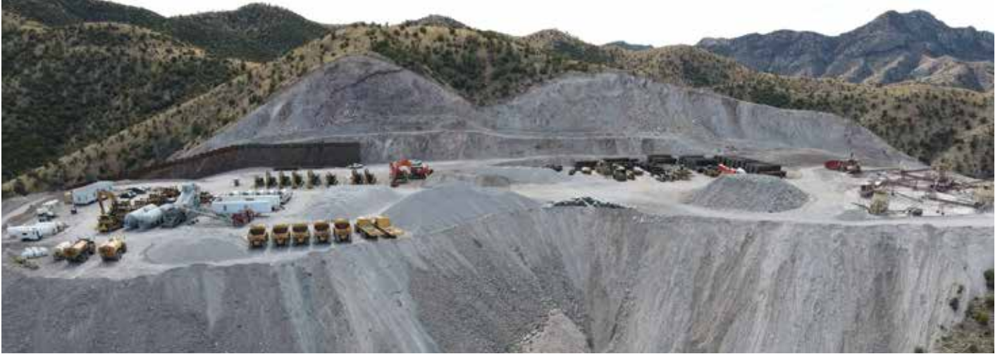
Drone photo looking south at Fisher Sand & Gravel Staging area 6 miles west of Nogales, Arizona. Coronado National Forest: Mar. 4, 2021. 31.3364, -111.077564. Photo: Myles Traphagen
