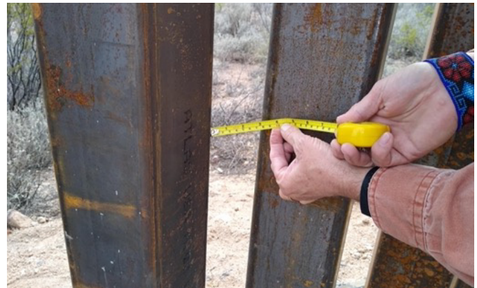
There are currently four inches between each bollard. Photo: Myles Traphagen
