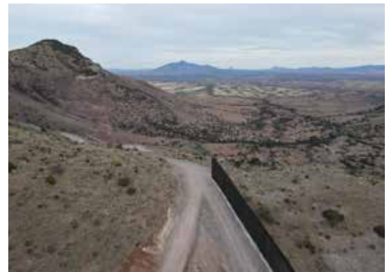
200-meter long "orphan wall" on west slope of Coronado Peak. Photo: Myles Traphagen
