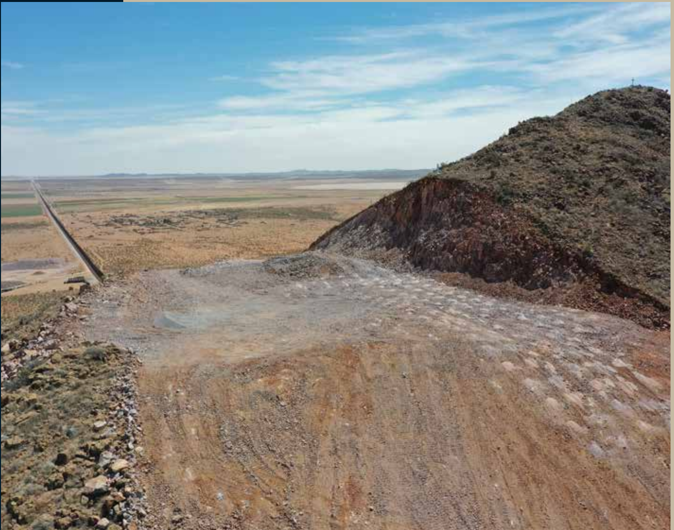
Dynamite blasting and mountaintop removal of Carrizalillo Hills, Luna County. Photo: Myles Traphagen
