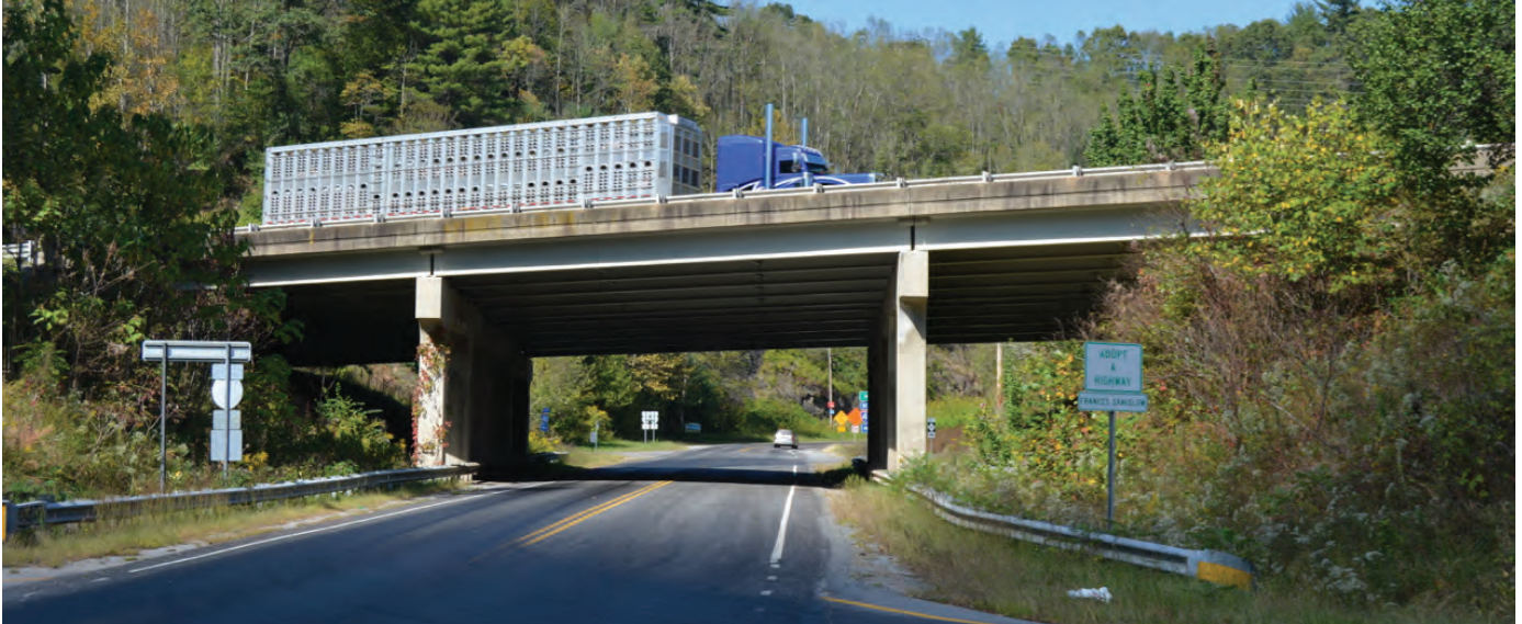
Fines Creek Bridge. Photo: Ron Sutherland
