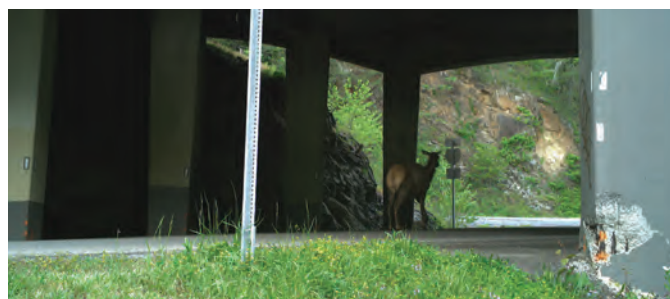
An elk uses the Waterville Bridge to pass under I-40. Photo: Wildlands Network / NPCA
