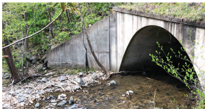
Fines Creek Culvert. Photo: Wildlands Network
