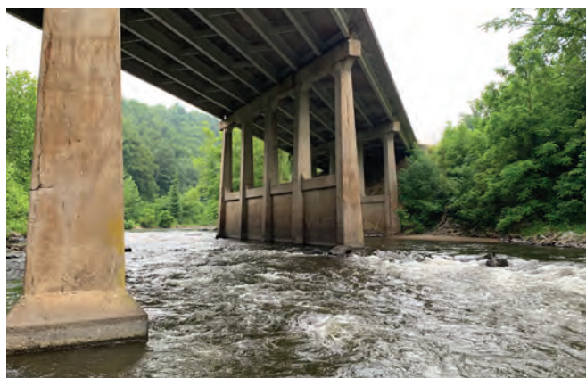
Pigeon River Bridge. Photo: Wildlands Network
