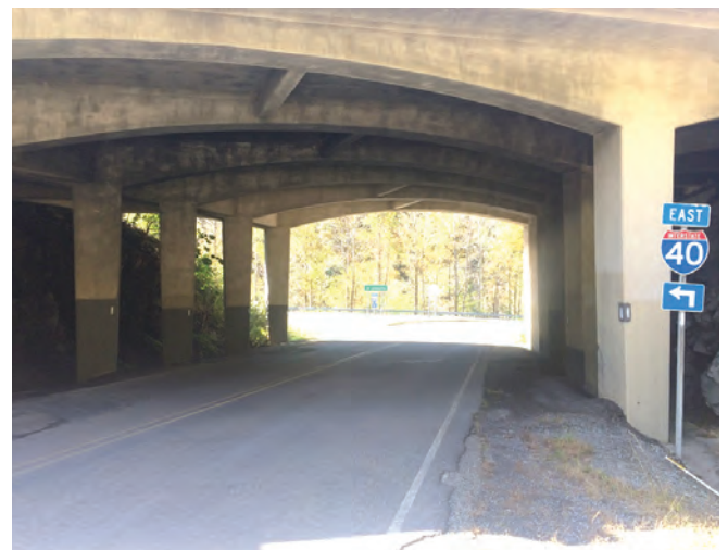
Waterville Bridge. Photo: Wildlands Network
