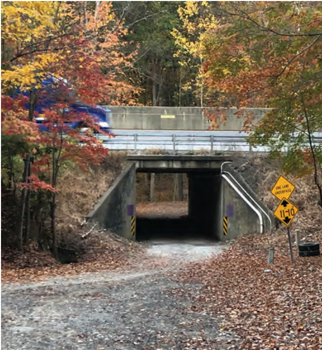
Wilkin's Creek Box Culvert A. Photo: NPCA
