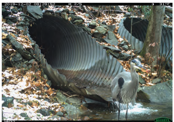
A great blue heron at the Groundhog Creek Culvert. Photos: Wildlands Network / NPCA
